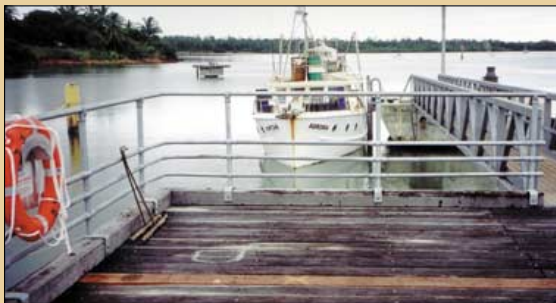
• SAFETY RAILS INSTALLED AT WEIPA.
