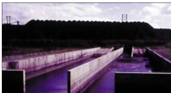
• A SETTLEMENT POND WHICH COLLECTS COAL RUN-OFF FROM STOCKPILES.
